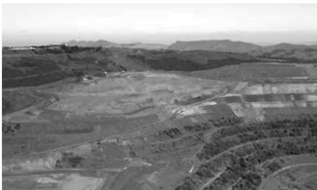
Dry disposal area
