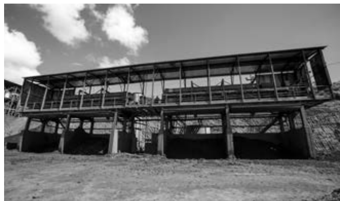
Installation of press filters
